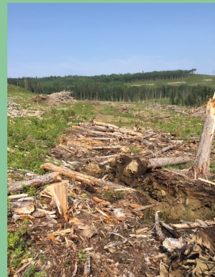
This photo above is looking along a road that had been rehabilitated following harvest the previous season. Cutting across the middle of the photo is a depression with a small watercourse; as shown from the intact vegetation the snow-fill crossing minimized impact to the riparian area. The road was rehabilitated and obstructed with debris, as shown in the photo below, to reduce hunting pressure on moose, based on a commitment made to First Nations.
