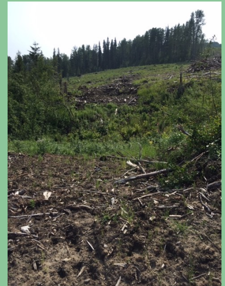
This photo above is looking along a road that had been rehabilitated following harvest the previous season. Cutting across the middle of the photo is a depression with a small watercourse; as shown from the intact vegetation the snow-fill crossing minimized impact to the riparian area. The road was rehabilitated and obstructed with debris, as shown in the photo below, to reduce hunting pressure on moose, based on a commitment made to First Nations.
